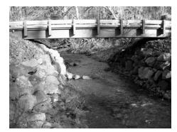
The bridge above on Green Diamond forestland was installed as part of the company's RMAP work. It was designed and constructed by modern engineering standards to address the issue of maintaining the stream's water quality and minimizing or eliminating sediment entering the stream. Green Diamond received a recognition award from the Shared Strategy for Puget Sound coalition for its proactive approach to road maintenance efforts and stream enhancement.
